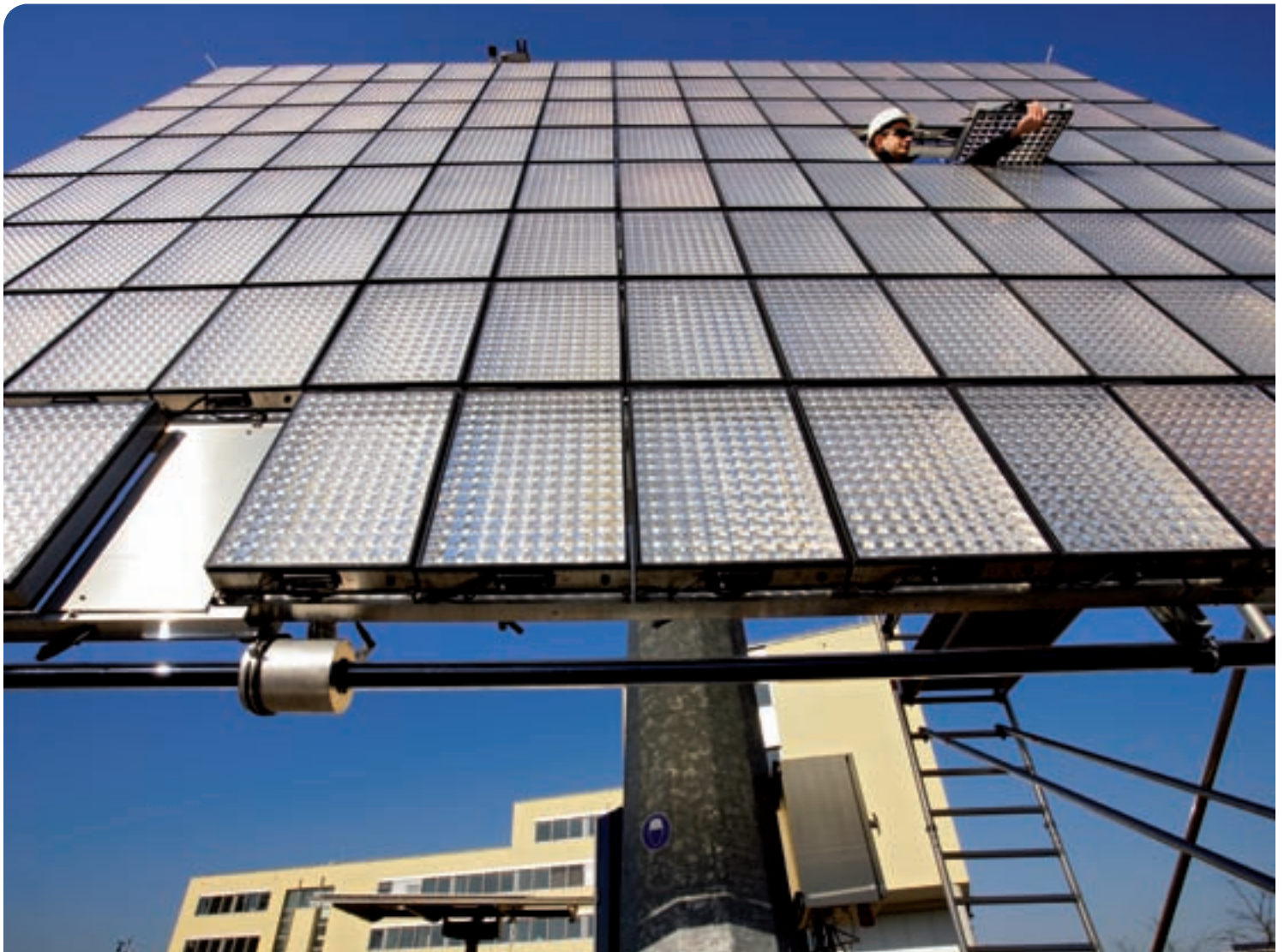
High concentration photovoltaic systems convert more sunlight into electricity than other solar technologies. © Concentrix
